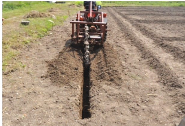
Field operation of prototype mini tractor operated trencher
